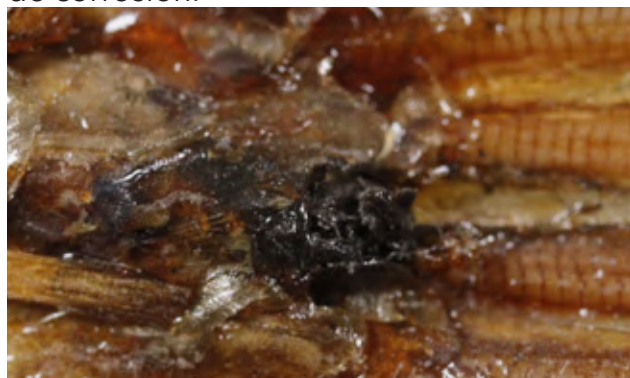
Fig.132 Armature interne corrodée visible
